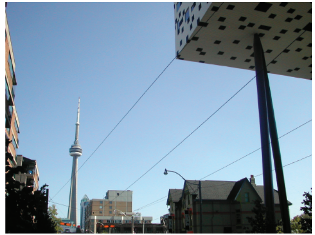
Figure 3: The slender columns as they taper at the point of contact with the underside of the building
