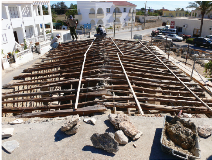
Exterior perspective of the Juniper beam used in roof construction
