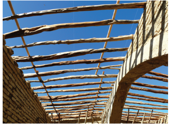
Interior perspective of the Juniper beam used in roof construction
